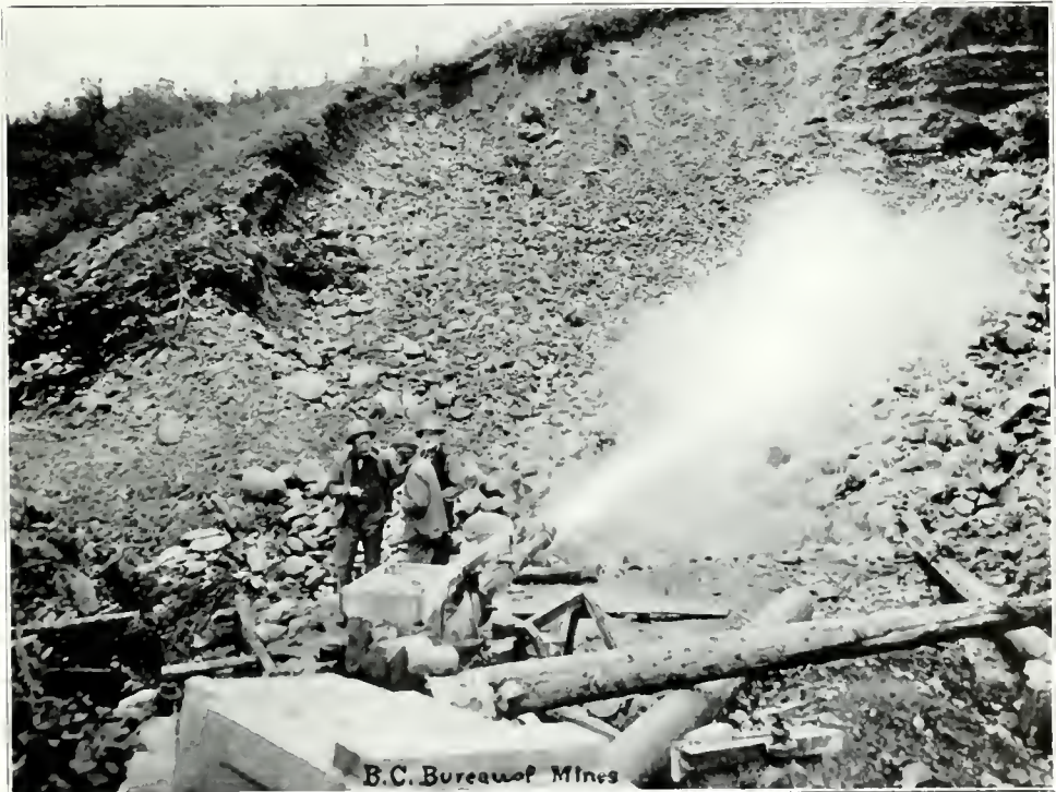
Opening Hydraulic Pit, Boulder Creek Mining Co.
